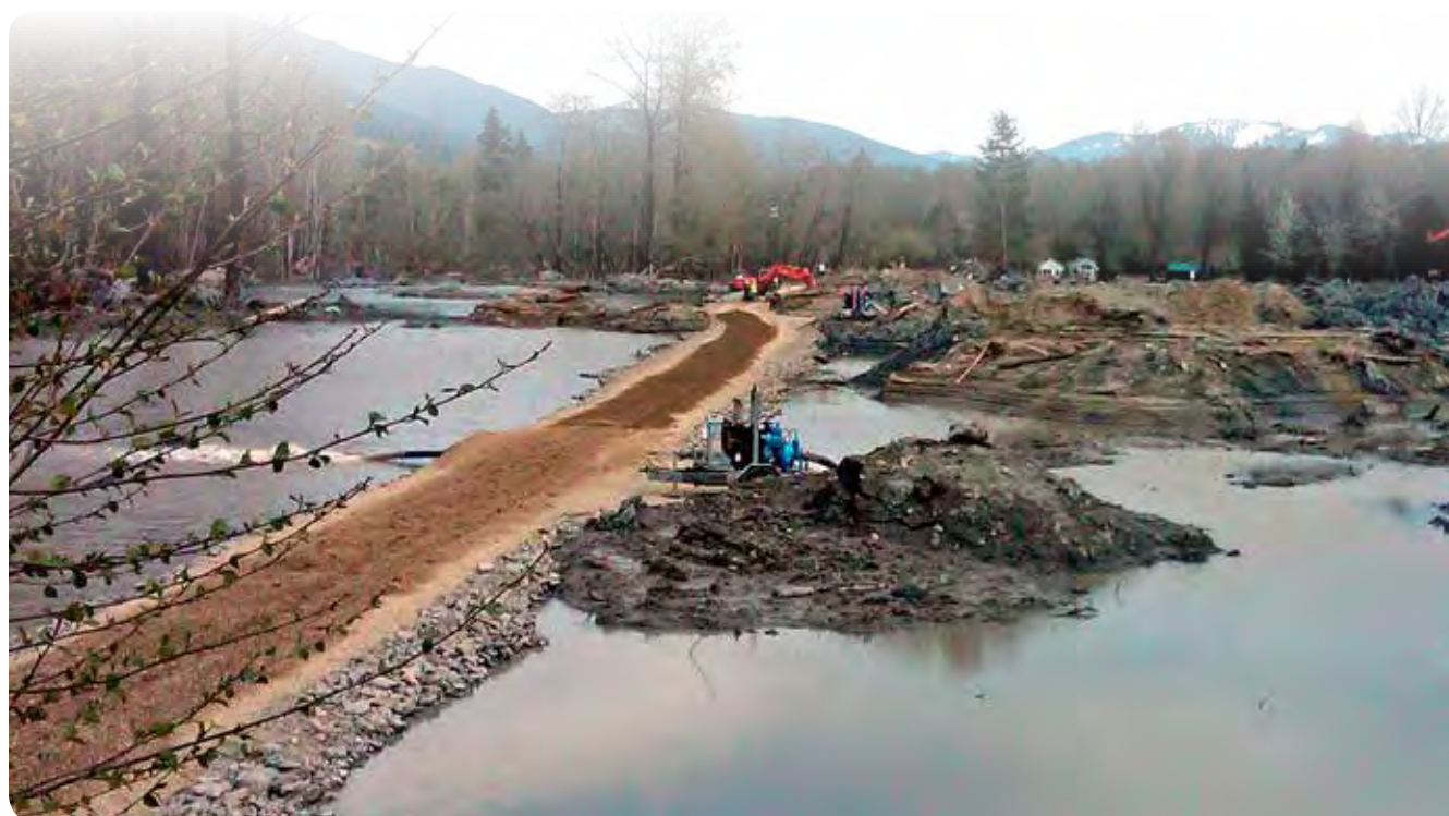
The U.S. Army Corps of Engineers, Seattle District, has nearly completed construction of the temporary berm within the SR530 slide area. (Photo courtesy of U.S. Army Corps of Engineers)
