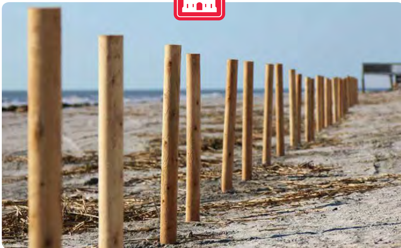
The Charleston District has begun the fencing and grassing project at Folly Beach to build dunes behind the recently completed renourishment project. (Photo by Sara Corbett)
